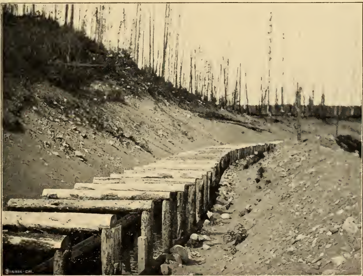
SHOWING DITCH THROUGH BAD GROUND. 43RD COMPANY'S FLUME AND DITCHES—OMINECA M. D.
